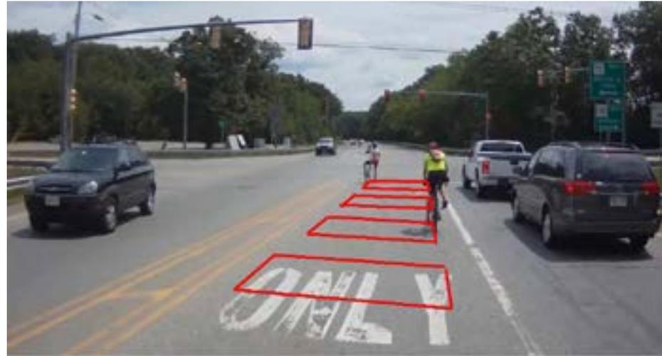
**Location of traffic-signal actuator loops at the left-turn from Route 140 to Route 70 on the Climb to the Clouds ride. The pavement cuts were visible. If enough cyclists lined up over the wires, the light would probably change. Screen shot from John Allen's video; artwork by Bob Shanteau.**
